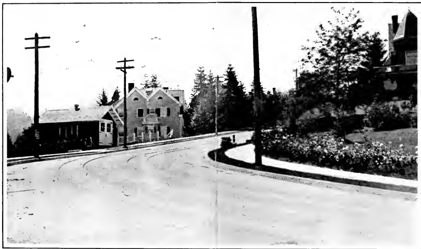
Hassam Pavement, Vista Avenue, Portland, Oregon. The portion of the street occupied by the streetcar tracks is also paved with 'Hassam'
